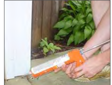
Seal holes on exterior of your house.
